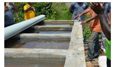
Farm water filtering system
